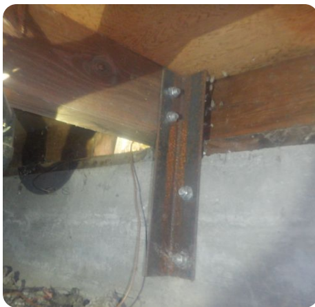
Supplemental angle iron straps securing foundation and framing.
