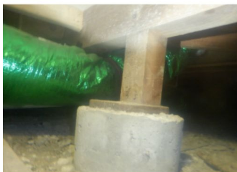
Post & pier construction within crawl space.
