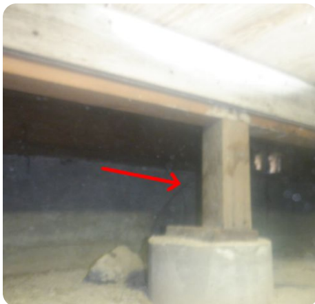
Post & pier construction within crawl space.
