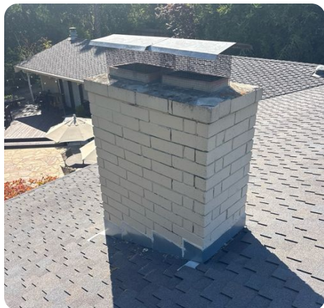
Functional chimney structure as viewed from roof surface.
