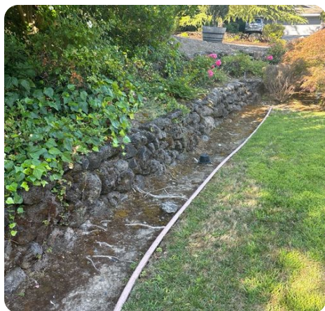
Functional stacked stone retaining walls.
