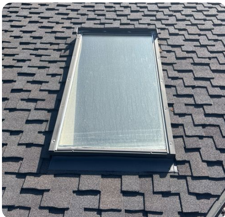
Functional skylight as viewed from roof surface.
