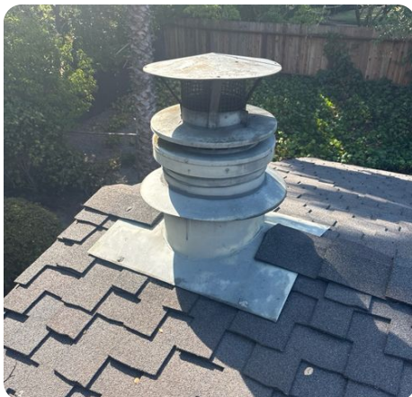
Fireplace chase cap as viewed from roof surface.
