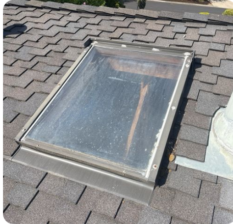
Functional skylight as viewed from roof surface.
