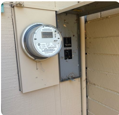
Original main service panel at garage exterior.
