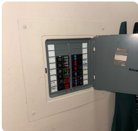
Original interior sub-panel within kitchen pantry.
