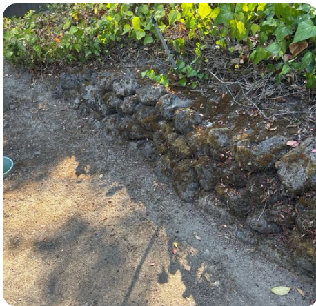
Functional stacked stone retaining wall.
