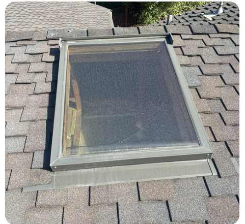
Functional skylight as viewed from roof surface.
