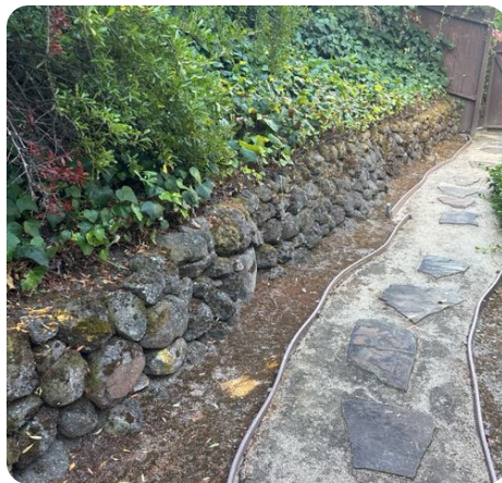
Functional stacked stone retaining wall.
