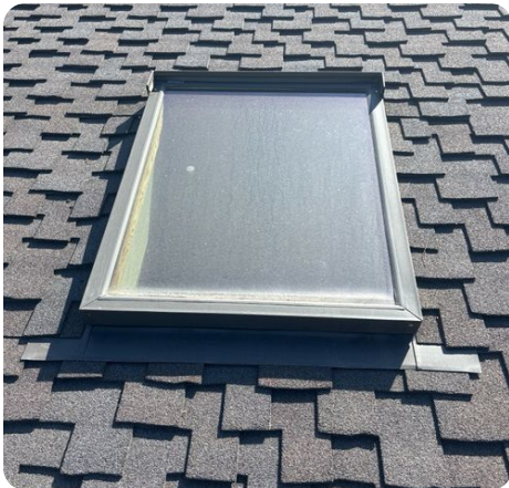
Functional skylight as viewed from roof surface.
