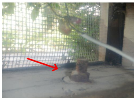
Sill plate anchor within crawl space.
