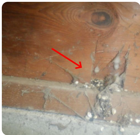
Sill plate anchor within crawl space.
