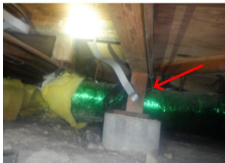
Post & pier construction within crawl space.
