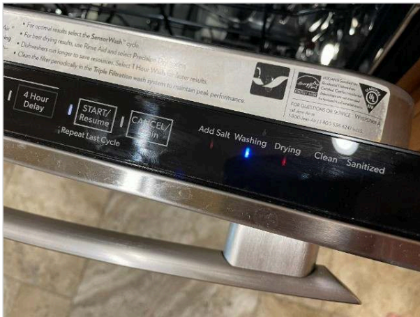
Blinking lights on this model indicates problem with dishwasher.
