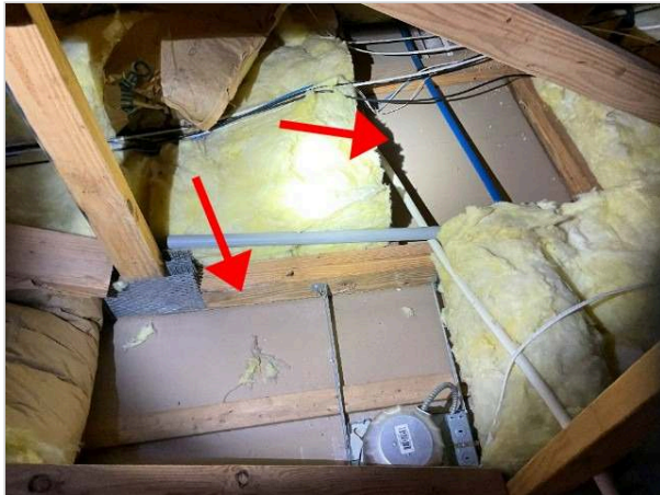
Missing insulation.
