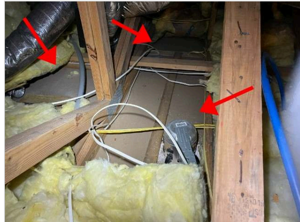
Missing insulation.
