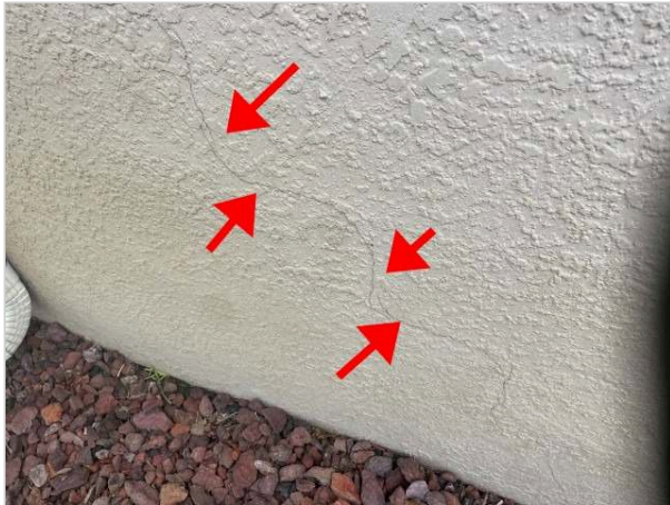
Minor crack.
