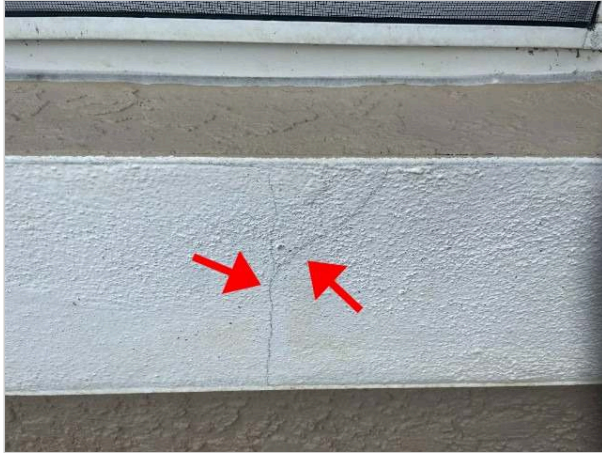
Minor crack.
